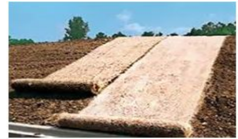
Erosion blankets/ coco-matting
