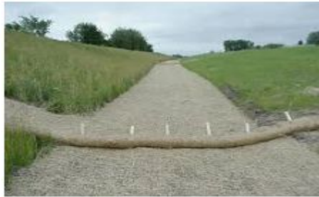
Sediment log (large & tightly packed) Wattle (smaller and loosely packed)
