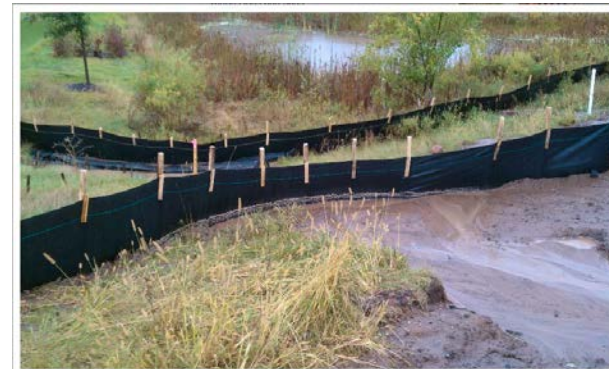
Silt fence/ filter cloth
