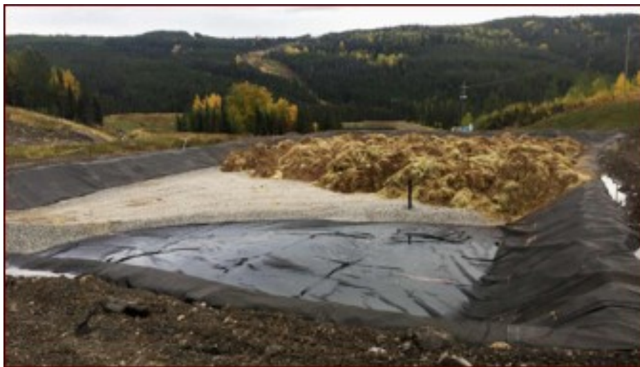
Photo 2. Reconstruction of BCR treatment cell, establishment of overlying substrate layer. 2017.
