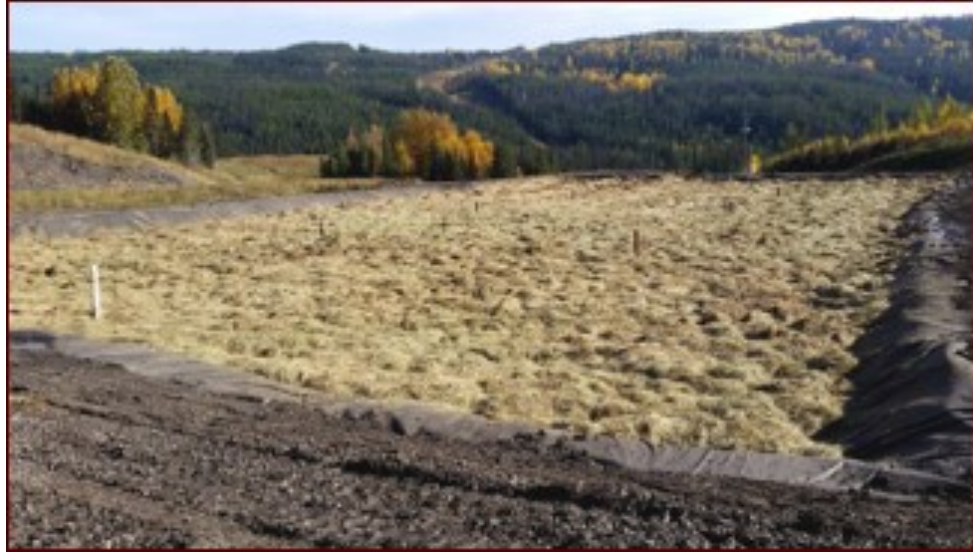
Photo 3. Reconstruction of the BCR treatment cell, with full substrate layer. 2017.
